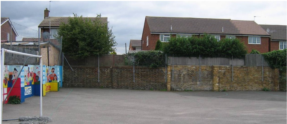
2. View of part of application site and southern boundary
